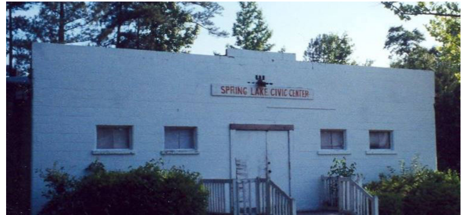
The Spring Lake Civic Center is currently being renovated as a space for the Sandhills Family Heritage Association. Plumbing and handicap access are the projects the group is currently fundraising for. (Photos courtesy of Sandhills Family Heritage Association Facebook page)
